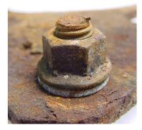
The **ATF/Acetone mix** is a 'home brew' you can make yourself with a 50-50 mix of automatic transmission fluid and acetone (nail polish remover). This removes tight nuts better than any commercial brand .
